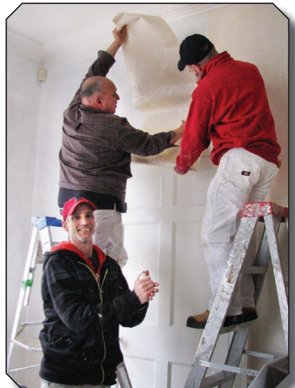
Below: An enthusiastic crew hangs wallpaper.
